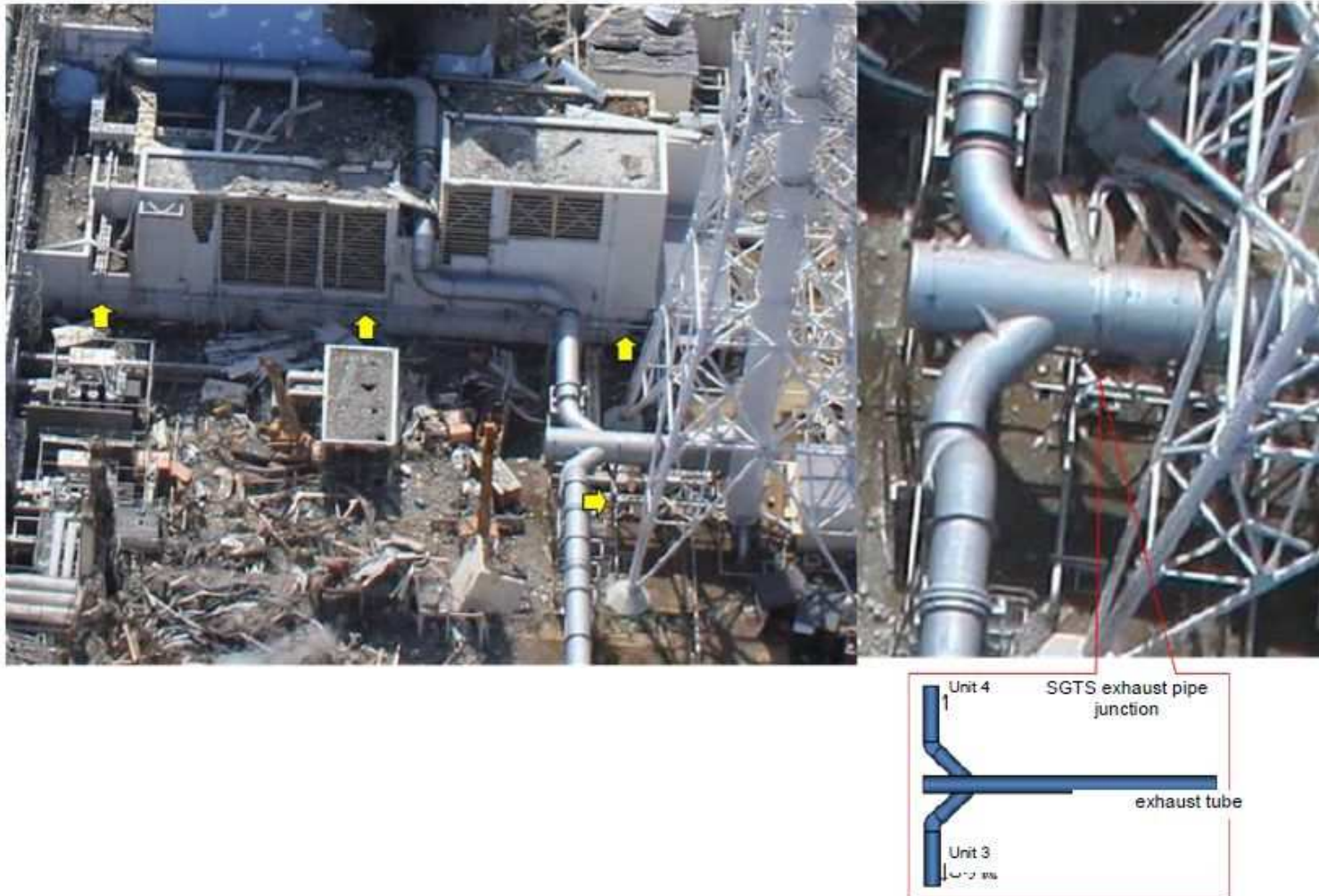
Fig. IV-5-11 Standby Gas Treatment System exhaust pipe
